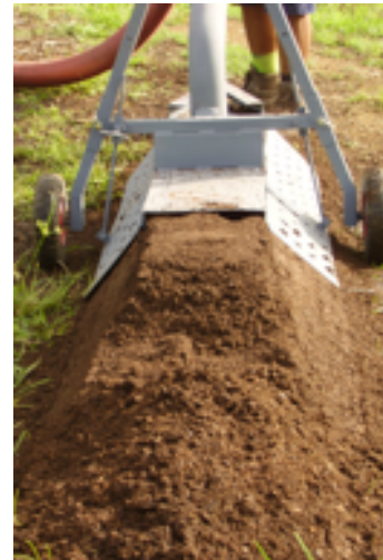
Inset: Construction of Reveg Berm
