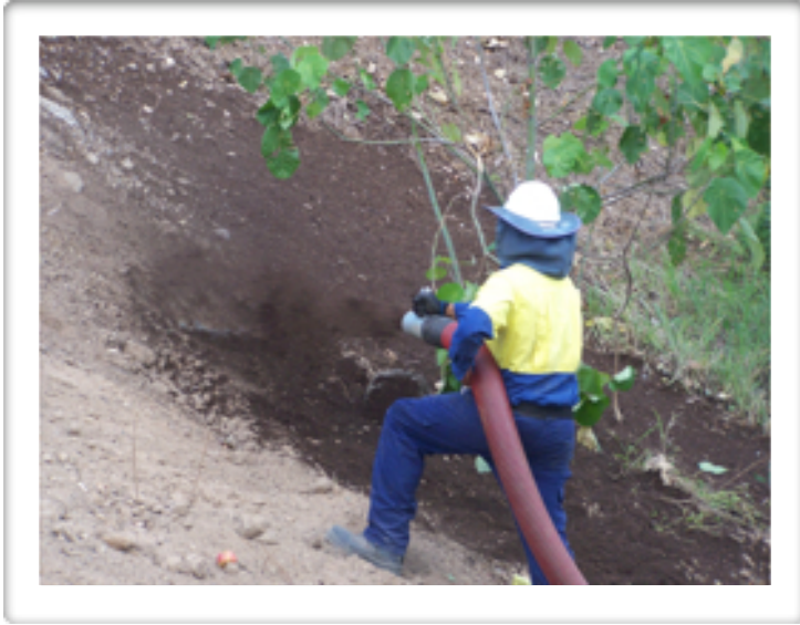
Photo: R.O.B being applied by the 'Reveg Express Bark Blower'.
