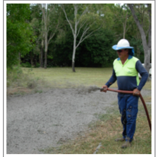
Photo: Hydromulch application
