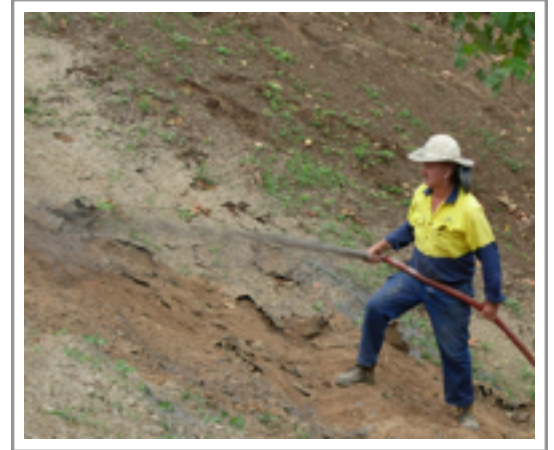
Photo: Bonded Fibre Matrix being applied.
