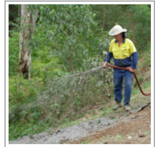
Photo: Bonded Fibre Matrix being applied from adjacent angle.
